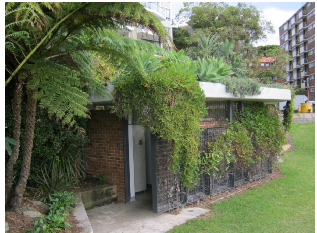
Roof garden and green walls at Beare Park public toilet
