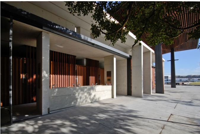
Pirrama Park public toilet – clear entrances open to active open space with absence of loitering cues.
