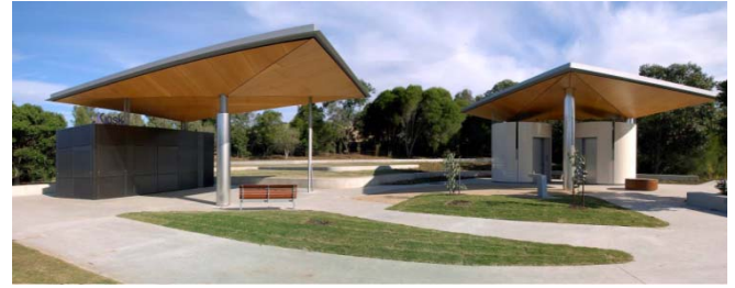
Public toilets at Sydney Park located adjacent café kiosk
