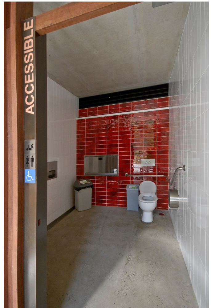
Pirrama Park toilets illustrating good practice inclusive access, large internal circulation space, and inclusive fittings and fixtures.
